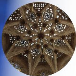
The lantern tower
